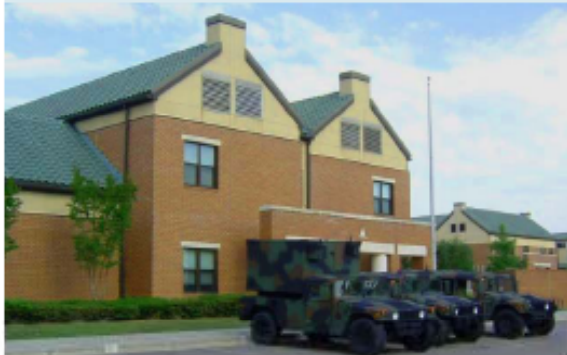
Fort Bragg Airforce Base, USA (Exhaust)
