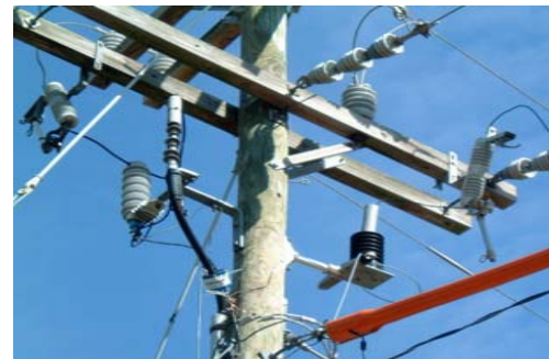
Coupler installation (overhead)
