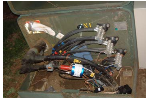
Coupler installation (underground)
